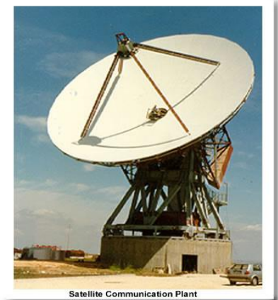
Small text caption below the satellite dish image: Satellite Communication Plant
